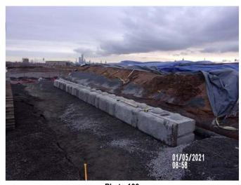
Photo 100 Installing Redi-Rock wall
