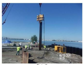
Photo 40 Installing temporary excavation support sheet piles
