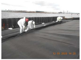
Photo 84 Stitching gas venting layer (GVL) panels together
