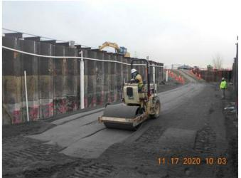
Photo 72 Backfilling and compacting structural fill within the Deferred Area
