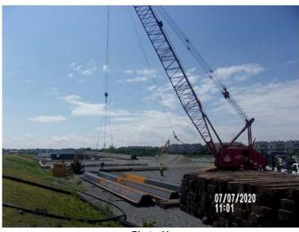
Photo 11 Unloading sheet pile on SA-6 South
