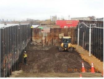
Photo 68 Installing lean clay along hydraulic barrier wall and placing common borrow in 1' lift within the Deferred Area
