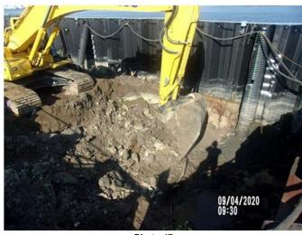
Photo 47 Excavating hazardous soil
