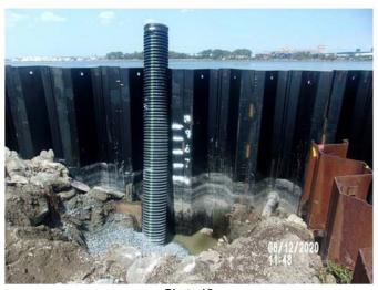
Photo 15 Installing dewatering sumps in the Deferred Area
