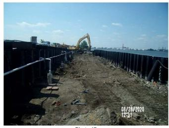
Photo 17 Installing depressurization wells, observation wells, header pipe, and electrical conduits for dewatering system inside the Deferred Area
