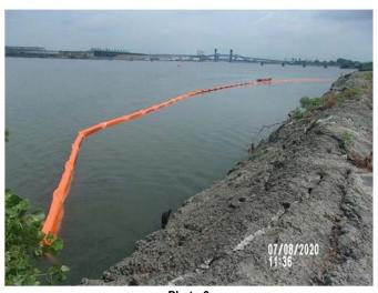
Photo 9 Installing and anchoring turbidity curtain
