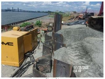
Photo 24 Installing reinforced hydraulic barrier wall
