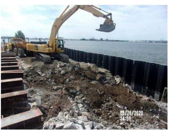
Photo 42 Removing concrete from the Deferred Area
