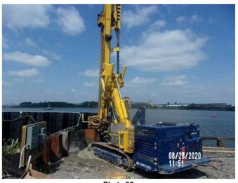
Photo 36 Installing grout columns
