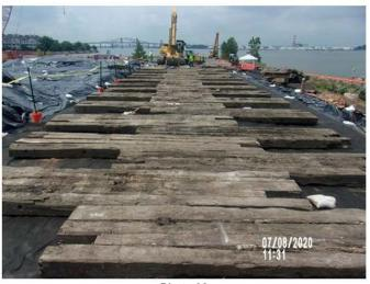
Photo 32 Constructing crane platform
