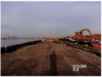
Photo 102 Installing lightweight fill in the Deferred Area
