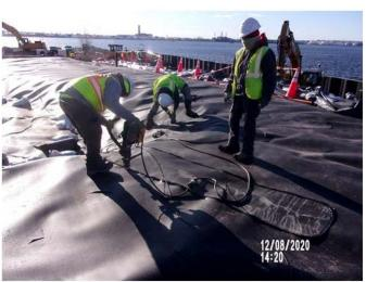
Photo 90 Extrusion welding repairs on LLDPE liner
