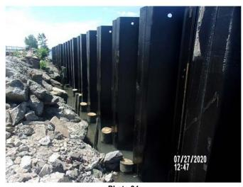
Photo 34 Installing permanent sheetpile along bulkhead
