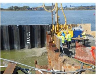
Photo 39 Jet grouting at north end of the Deferred Area
