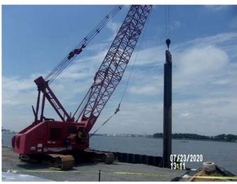
Photo 33 Installing permanent sheetpile along bulkhead
