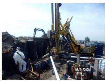
Photo 16 Installing depressurization wells
