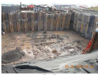
Photo 52 Bottom of Excavation Area 2 (-3.3 ft)
