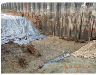
Photo 57 Bottom of Excavation Area 1C-2 (-10.2 ft)
